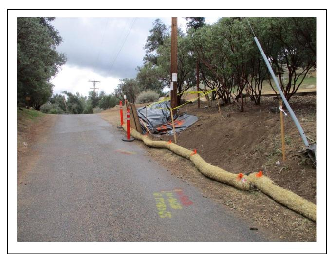
**Photo 5:** At P178056 (C 442), dirt spoil was covered and fiber rolls were in place to prevent erosion in accordance with the Erosion Control Plan and SWPPP. The pole hole was securely covered for safety and to prevent wildlife entrapment in accordance with MM-BIO-23.
