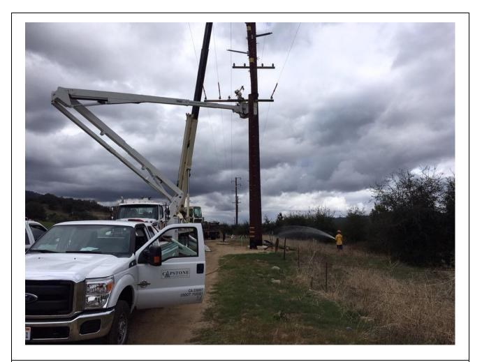
**Photo 4:** During cutting of the existing steel distribution pole at Z118048 (TL 682), a fire patrol was observed monitoring the hot work and wetting down the surrounding area in accordance with the CFPPP.
